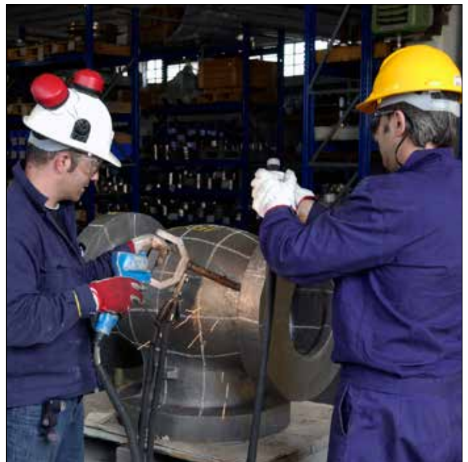
MAGNETIC PARTICLE INSPECTION
